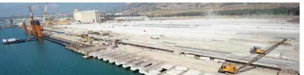
Under Çandarlı Port Breakwater Construction Project carried out by the Joint Venture Group of Limak and Kolin, a breakwater with a total length of 1.800 m, of which 800 m involve stone fill and 1.000 m, steel pipe piling, and a dock with a total length of 2.000 m and a depth of 18 m are under construction.
