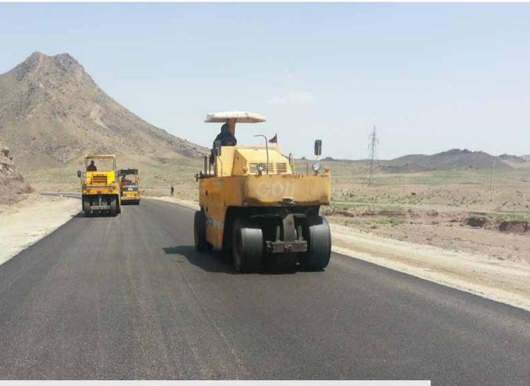
Highway No N-50 having a length of 531 km is a major highway linking Quetta, Capital of the State of Baluchistan to the State of Punjab in the north and further to Islamabad. Quila Saifullah - Zhob slice (ICB-3B) of this road is 150 km and built by the Joint Venture of Limak and ZKB JV. The dual carriageway road has a total width of 12,3 m.
